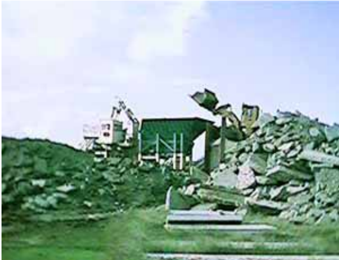
Concrete crushing operation
